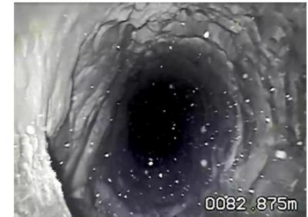
Figure 26: Cavity at a depth of 83 MBGL. Down view.
